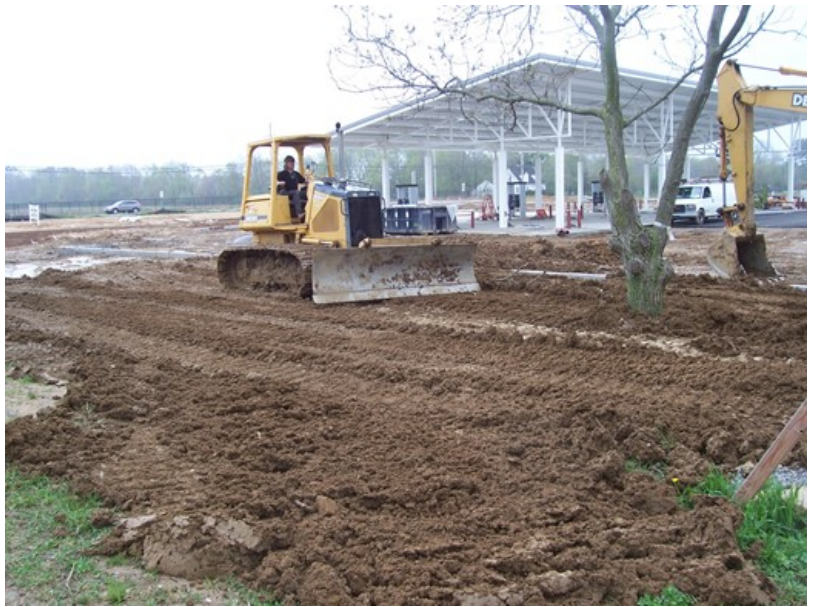
Figure 1. Soil compaction can occur during construction activities due to repeated operation of heavy machinery, especially when soil is wet.
