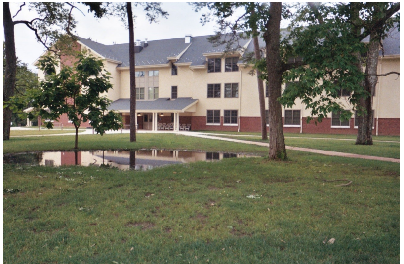
Figure 4: Water ponding on the surface of the lawn can show compacted soils that are inhibiting infiltration into the ground.
