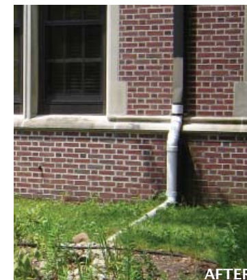
The image on the far left shows the approximate drainage area for a roof with more than one downspout. The two images in the center and near right depict both before and after the disconnection of the downspout from underground pipes.
