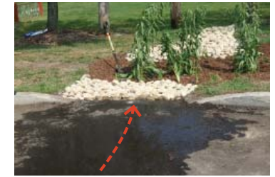
A curb cut and a stone buffer provides the inlet for runoff to enter the rain garden from the adjacent roadway.
